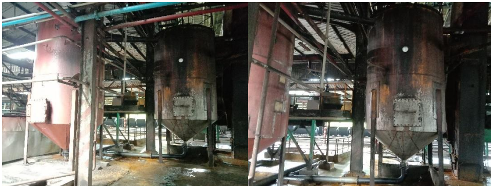
Gambar 3. 29 Sand Trap Tank
