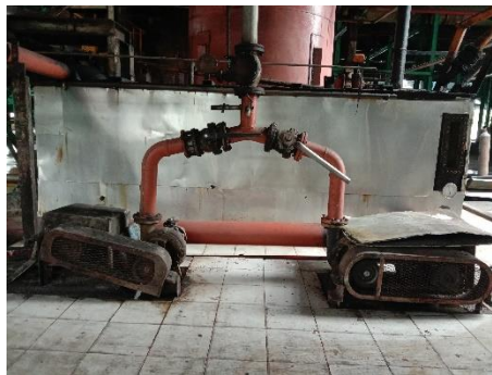
Gambar 3. 31 Crude Oil Tank
