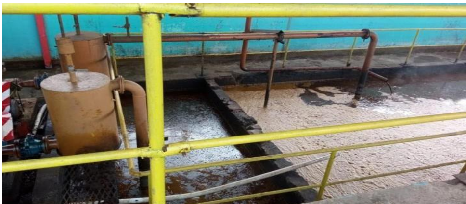
Gambar 3.33 Condensate pit
