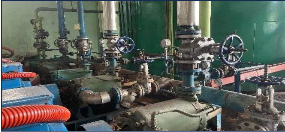
Gambar 5.10 Pompa Boiler
