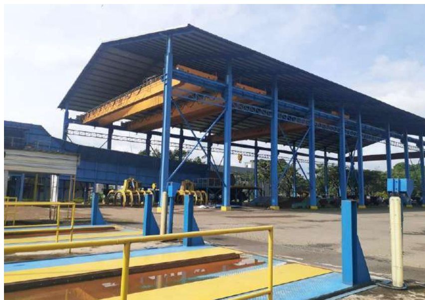
Gambar 2. Unit Overhead Cane Unloading Plus Tambahan Cane Carrier
