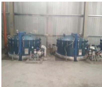
Gambar 3. 11 Niagara Filter
