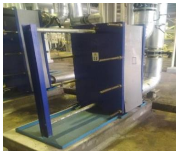
Gambar 3. 8 Plate Heat Exchanger
