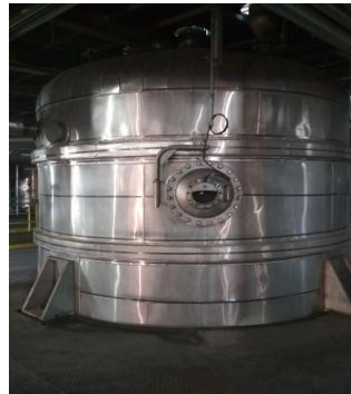
Gambar 3. 10 Bleacher Vessel
