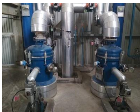
Gambar 3. 12 Filter Pulsetube
